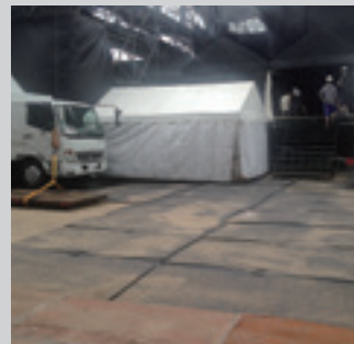
Event stage construction work
