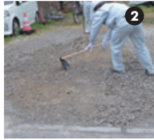
Level the ground
