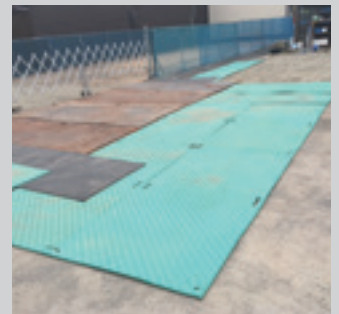
Construction site entrance
