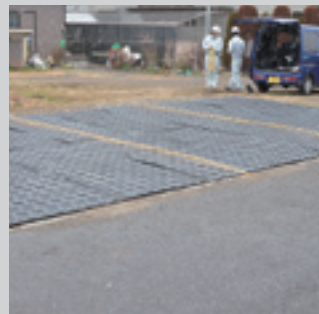
Temporary parking lot
